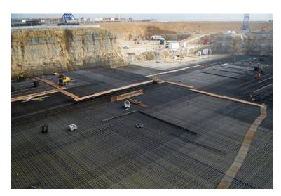
Steel reinforcement bars—each one weighing nearly 100 kilos—are built up to 1.5 meters on the floor of the Seismic Pit. In the distance, the future ITER Headquarters buildings rises above the platform. (August 2011).
